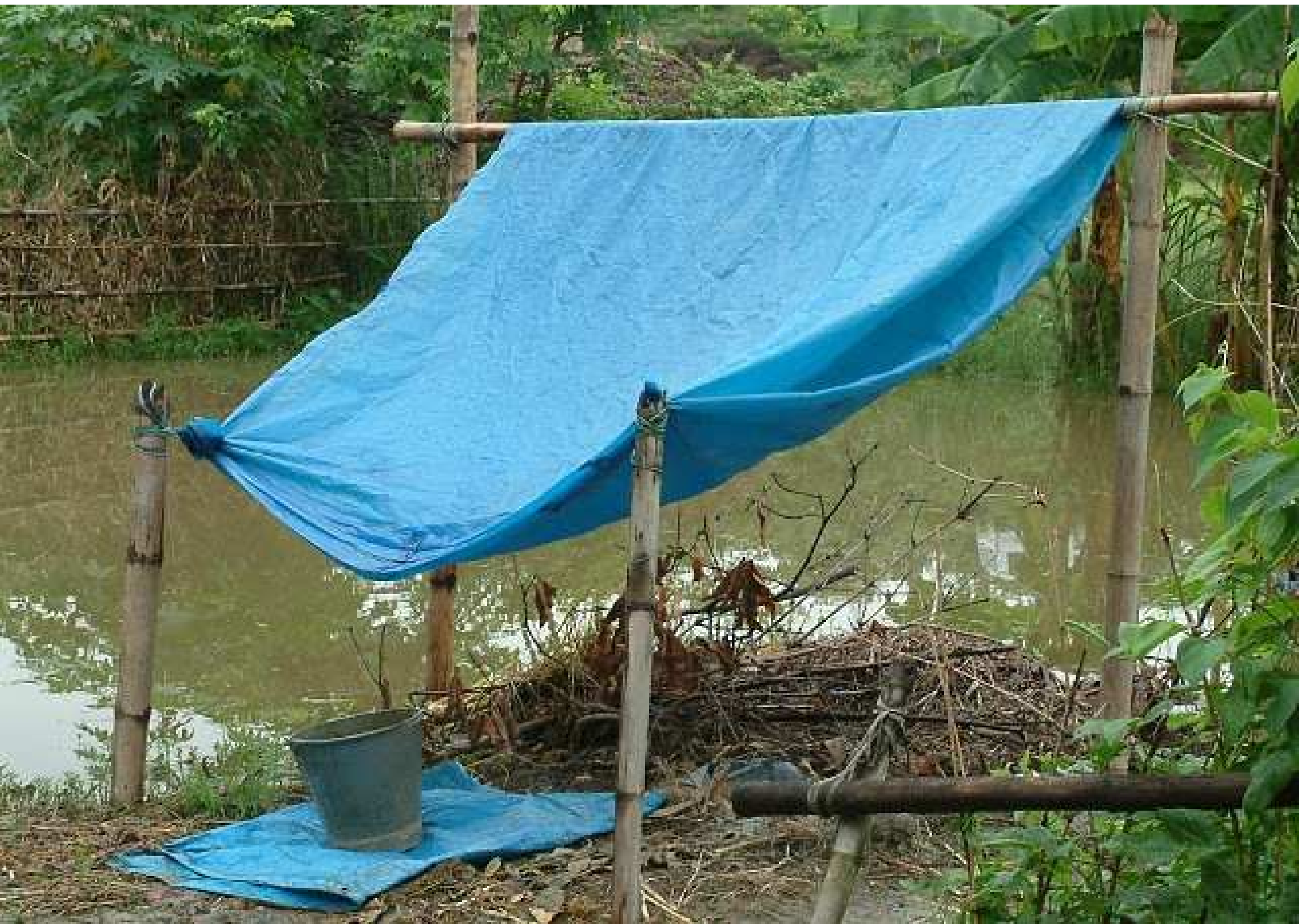
46. Textile rainwater collector
