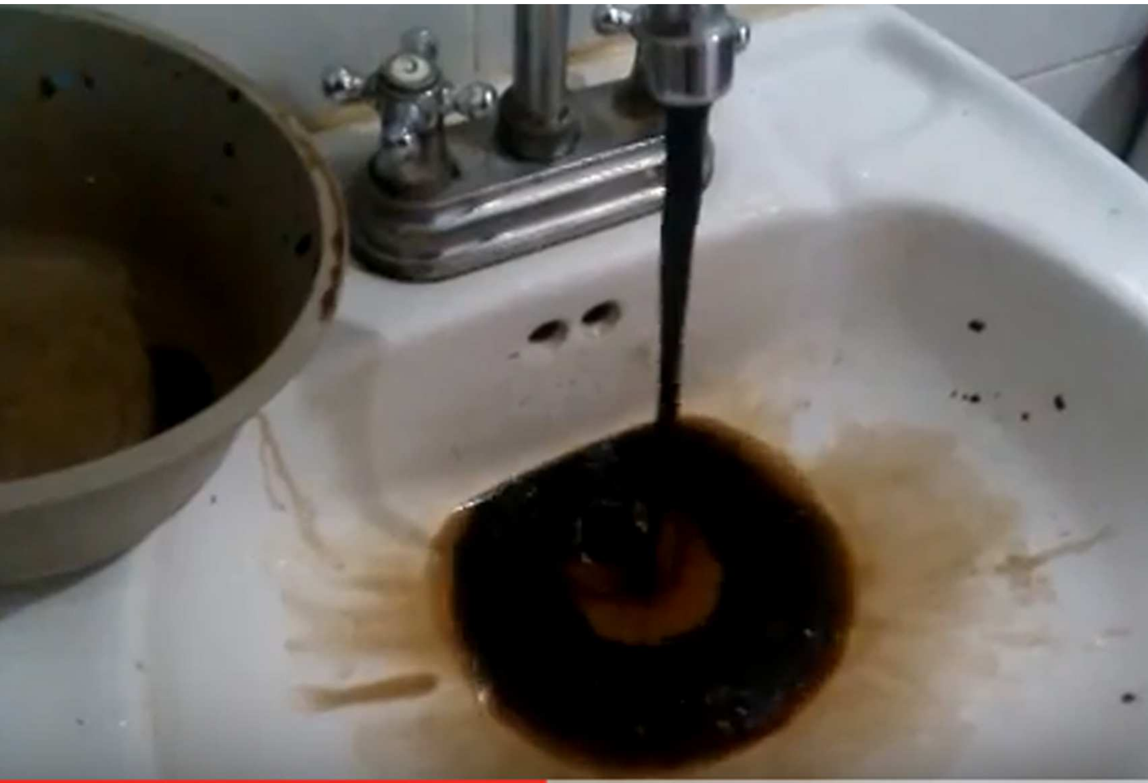
31. A domestic horror in Iztapalapa: black color water is running from drinking water taps
