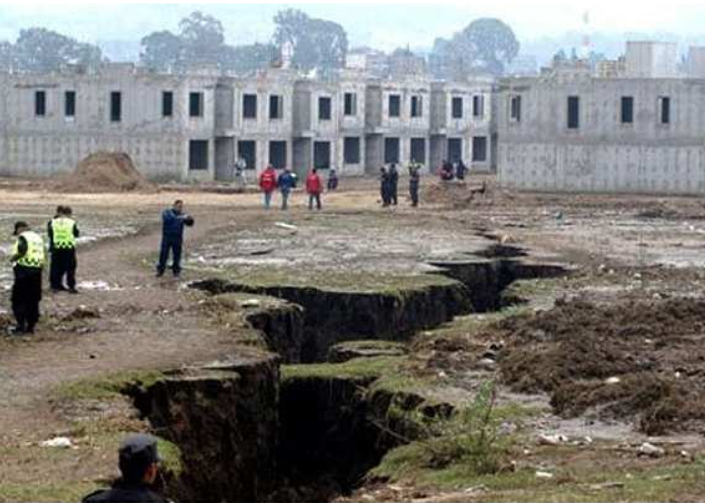
19. A huge land crack appeared in Santa Maria Huejoculco in Chalco, State Mexico in 2011
