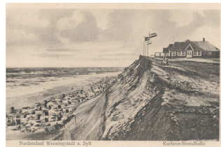
18 // Sylter hotel built on the cliff
