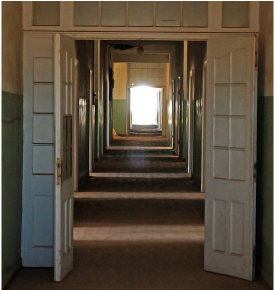
47 // Inside the hospital
