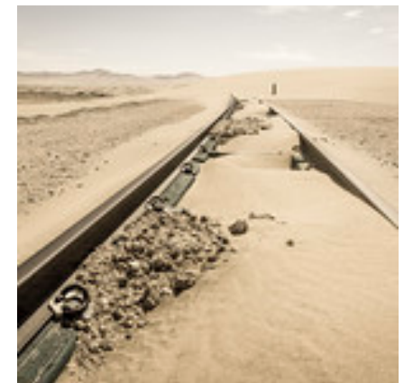
49 // Train tracks buried under sand
